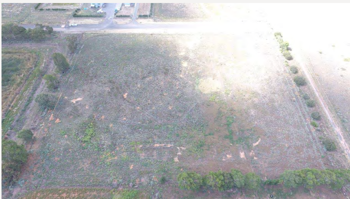
Figure 5 – Aerial view of Lot 1 looking north with dwelling demolished
